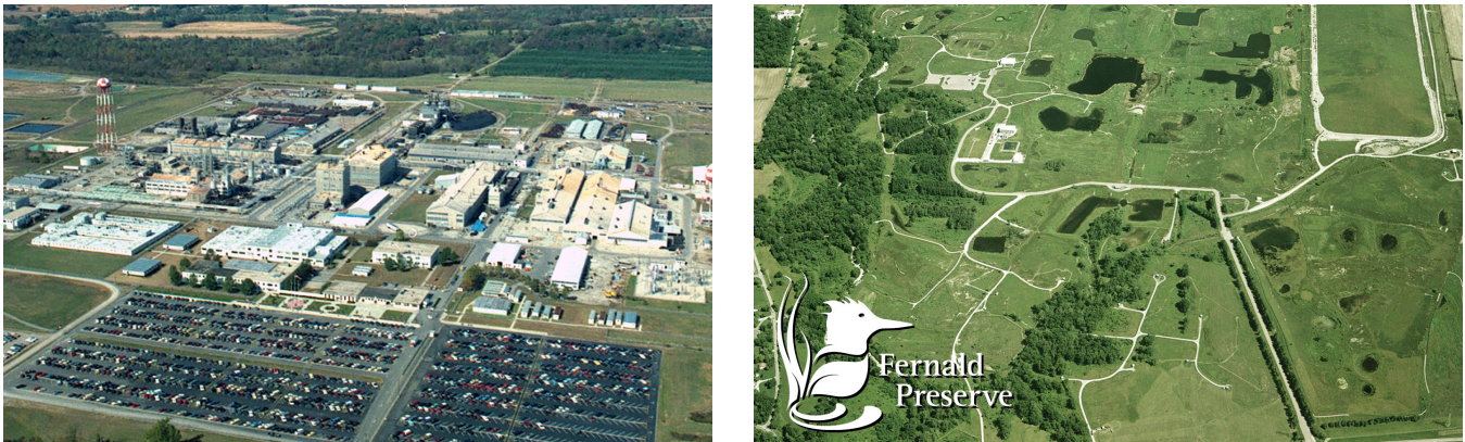
FIGURE 4: Fernald Site in 1987 (left) and 1990 (right). Photos courtesy of U.S. Department of Energy.
