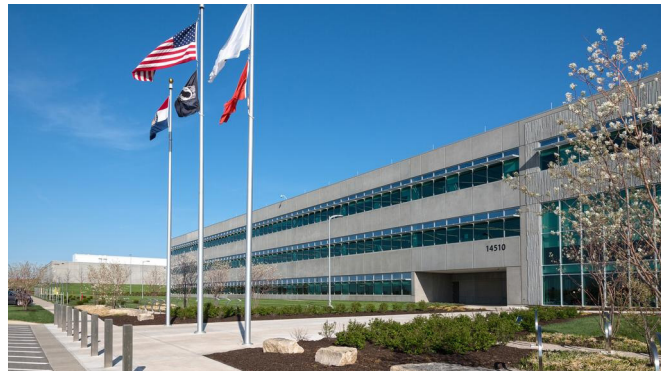
FIGURE 11: Kansas City National Security Campus. Photo courtesy of U.S. Department of Energy.
